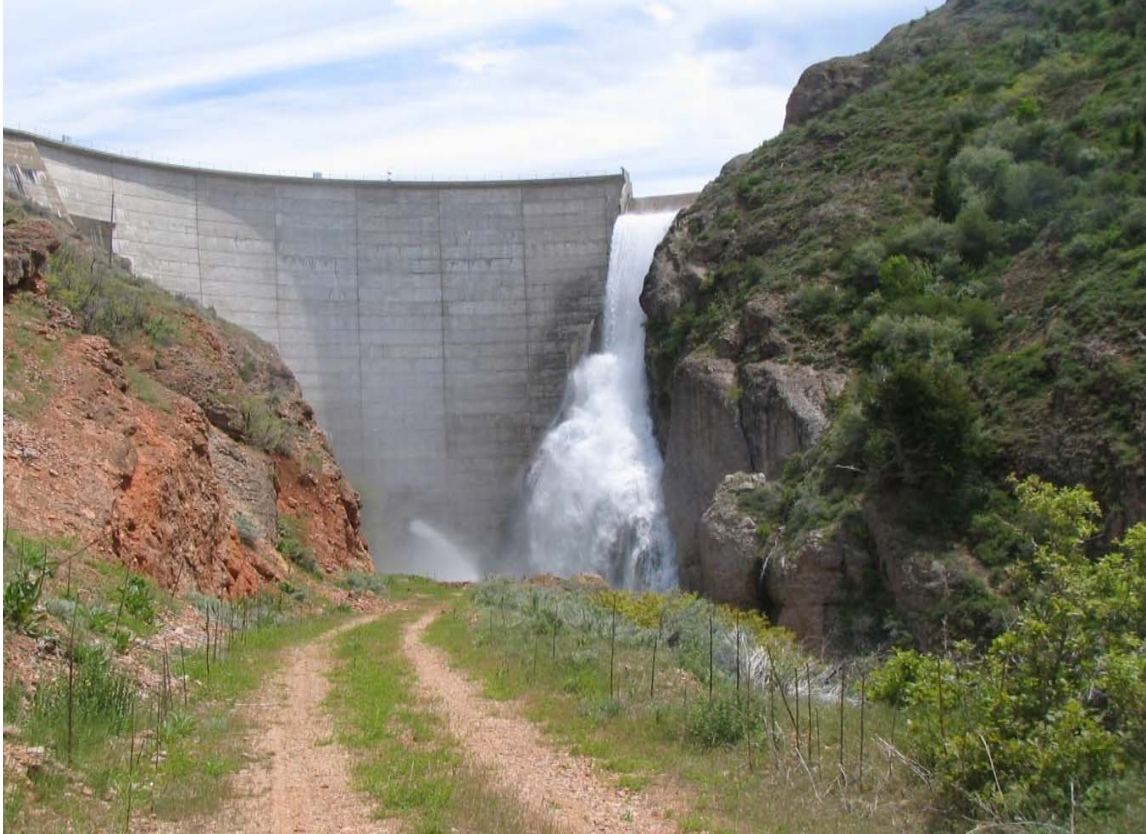
Figure 1.3.2-2 is a picture of East Canyon Dam spilling in June of 2008, (Provided by Nick Williams, USBR, 2008). Note the outlet discharge left bottom of spillway. Dissolved oxygen is reaerated to saturation at the outlet. This image also helps visualize the steepness of the reservoir and why so much of the storage capacity resides in the upper elevations of the reservoir. The surface spillway skims the warmest water from the epilimnion in June, and may also export spring algal bloom biomass.
